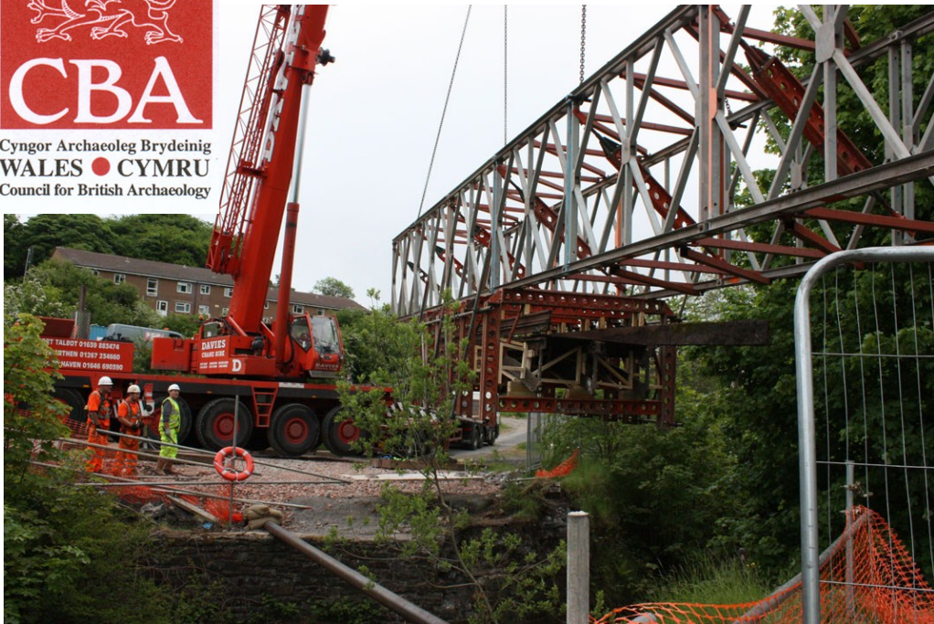
A flying Scheduled Ancient Monument! Aaron Brute's Bridge Blaenavon, in the process of being returned after conservation.
