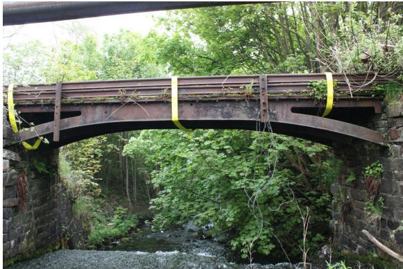
Bridge prior to restoration
