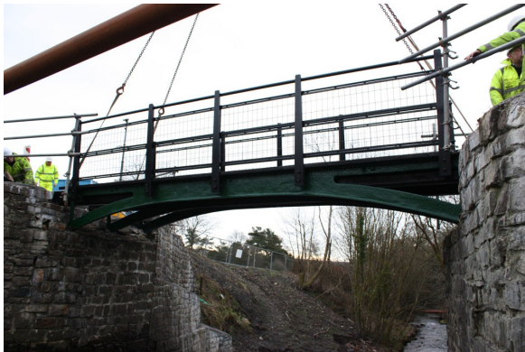
The restored bridge returned
