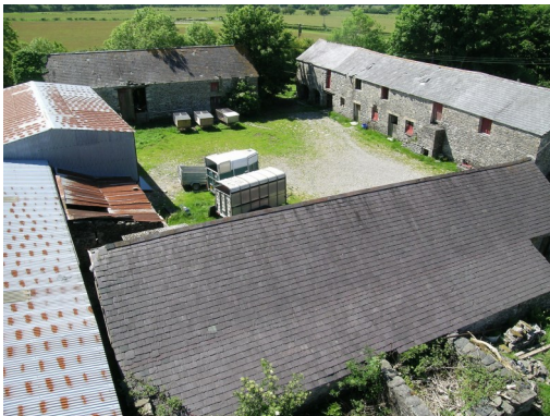
Strata Florida Farm courtyard
