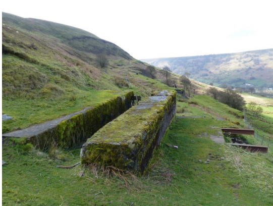
The Red Ash Level from the north
