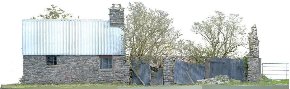
Figure 1: Tŷ Pair and cart shed west facing elevation prior to conservation
